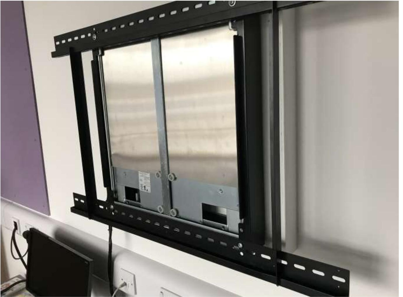
Photograph showing the Promethean Screen bracket after the screen has fallen.
