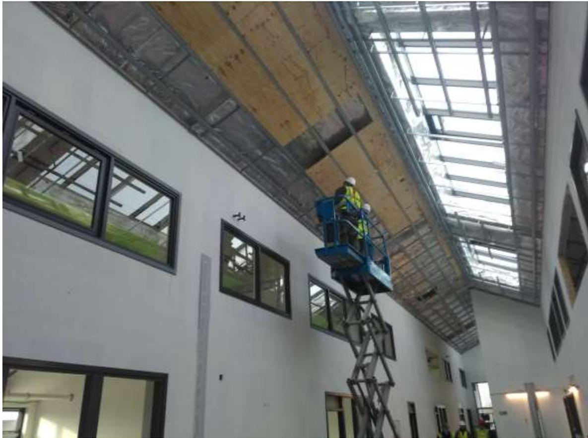
Photograph of ceiling install showing underside of cassette, MF ceiling rails and plywood pattrensing.
